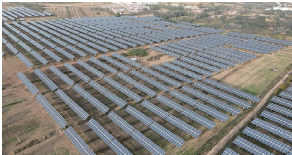
▲ Figure 9: Panorama of the demonstration power station
